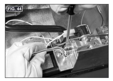
Connect wiring to the thermodisc on the flue jacket. This connection is not polarity sensitive. See FIG. 45.
