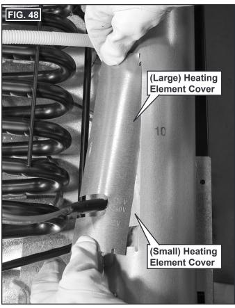
23. Lock (large) heating element cover to the flue jacket tab. See FIG. 49.
