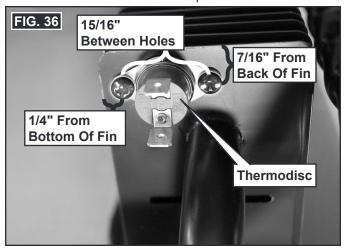
Cut the OLD 3/16" flag terminals off the thermodisc wiring, and replace with NEW 1/4" flag terminals. Connect the wiring to the thermodisc. This connection is not polarity sensitive. See FIG. 37.
