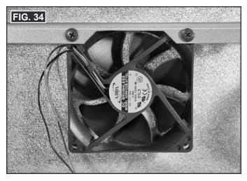
Place NEW fan bracket (with fan(s) mounted) under left side of cooling unit frame (near cooling fins) and over right side of frame. Align the mounting holes of the fan bracket to the cooling unit frame, and place and tighten the two mounting screws. See FIG. 35.
