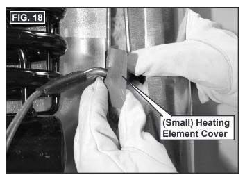
21. Remove heating element with (small) heating element cover by lifting up through the flue jacket's separated seam until it clears heating element pocket. Save heating element and heating element cover for reinstallation. See FIG. 19.
